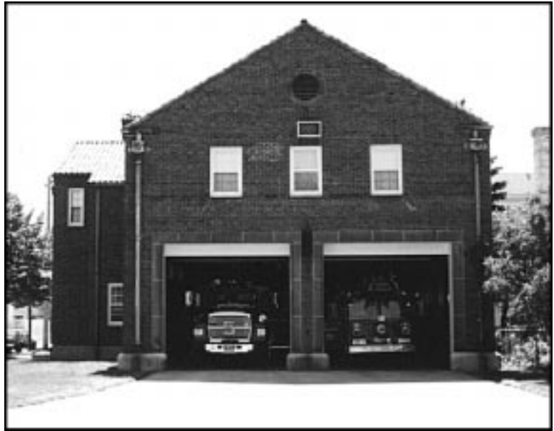
Station 5 (shown here in the 1980's) at the s.w. corner of Ashland Ave. and Victoria St. housed Engine 5 and Ladder 3 when it opened in 1930 on the former site of Chemical 6. The two companies moved from their former quarters at Selby Ave. and Makubin St.
