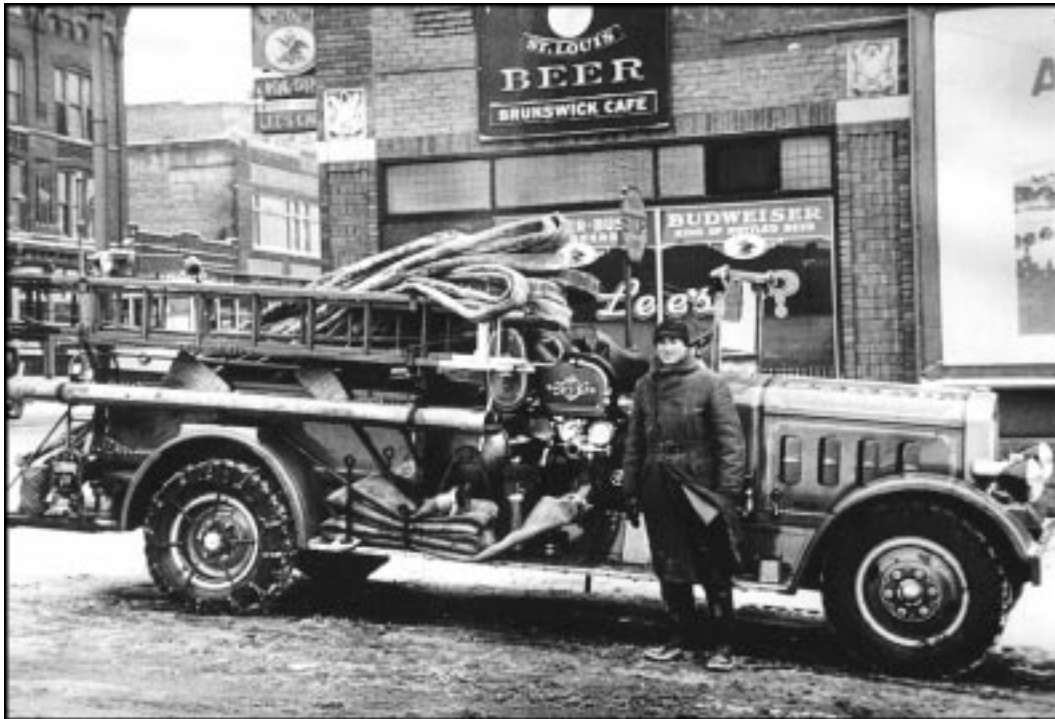
The 1933 Luerne 750gpm triple combination pumper is shown here as Engine 3 getting ready to return to quarters with a full load of frozen wet hose. The StPF D shops used the hose body is from the former 1913 American LaFrance Hose and Chemical and the Luerne chassis to construct the rig.
