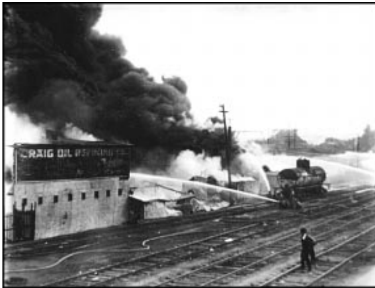
The Craig Oil Co. fire of May 19, 1924 (described in the previous chapter) at Morrison and Eaton Sts.
