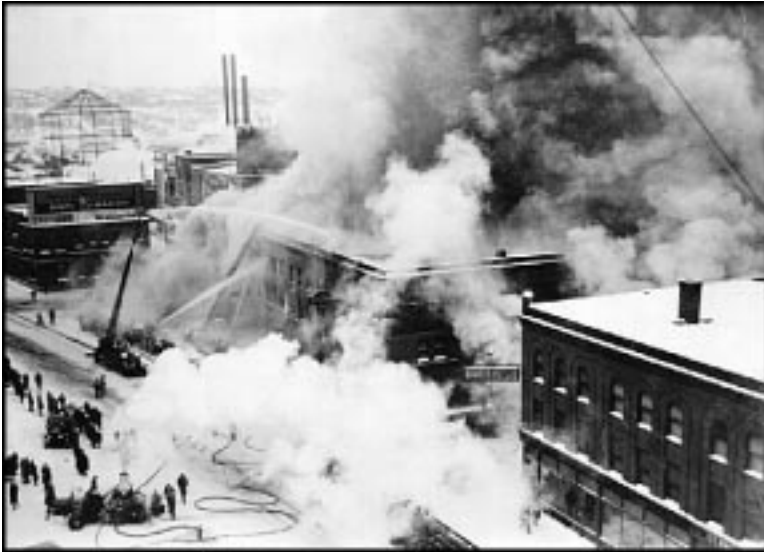
Another interesting shot of the "Commission Row" fire with a steam pumper in the foreground and Water Tower 1 playing a stream onto the roof of the buildings. The steamers certainly contributed to the smoke at the scene.
