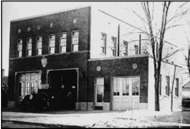
Station 7 on Ross just west of Earl St. opened in 1930. A small police precinct station was added on the west side of the station.
